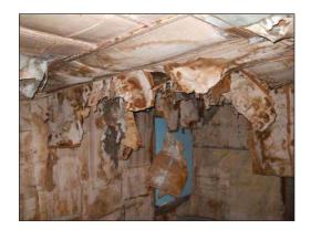
No south interior wall remains in the Coggswell Cabin to shelter it from the elements, and the protective muslin is clearly beyond repair with weather and water damage.
