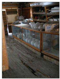
Figure 21: Charlie Bovey Building in desperate need of stabilization-floor is sunken in, endangering collections
