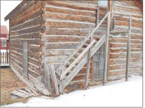
Figure 15: Rotting boards require consolidant
