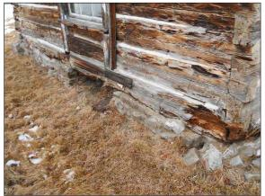
Figure 23: Failing foundations and rotting logs need to be addressed
