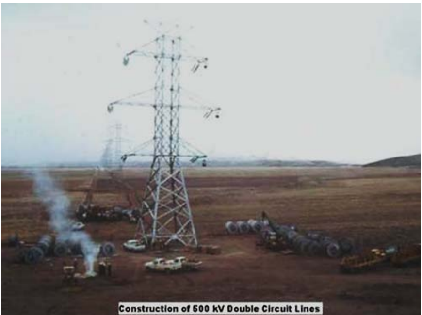
Construction of 500 kV Double Circuit Lines
