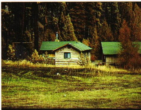
Impacted house in Laird creek immediately after the fires
