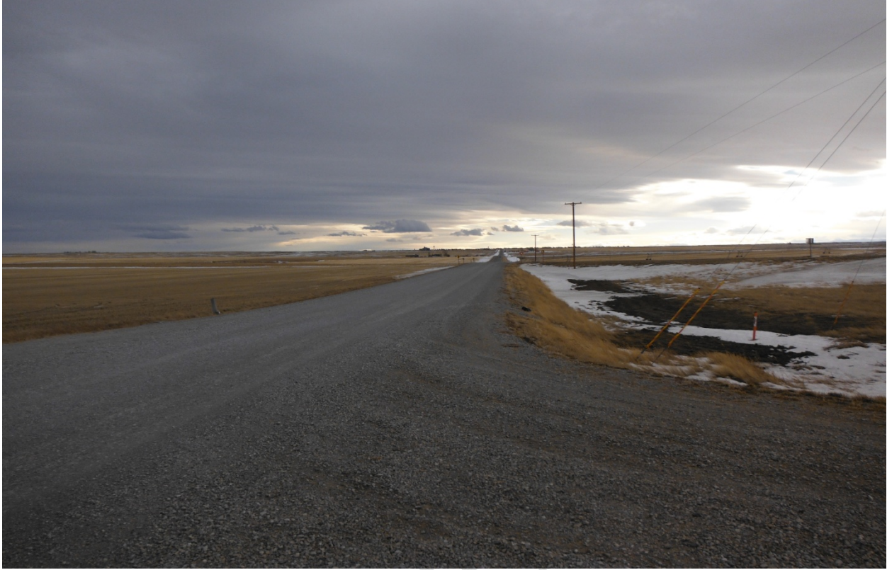
Route 358, Mile Post 3, 3 miles north of Valier, one leg of two-directional intersection. (400' X 16' road width)
