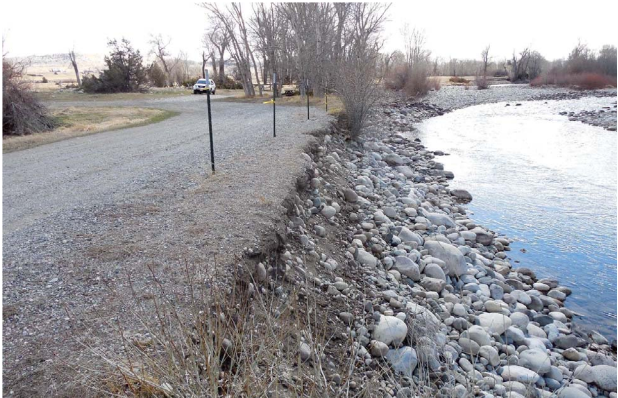
Photo 1. Loop Road Almost Undercut by Boulder River at Big Rock FAS
