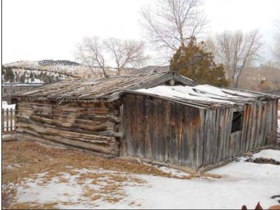
Figure 17: Rear portion of Richards Cabin collapsing- safety issue
