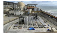
Dry cask storage at the San Onofre Nuclear Generating Station. Courtesy: Southern California Edison
