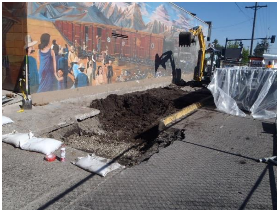
Removal of asbestos used as fill under a sidewalk, CMC Asbestos Bozeman Facility
