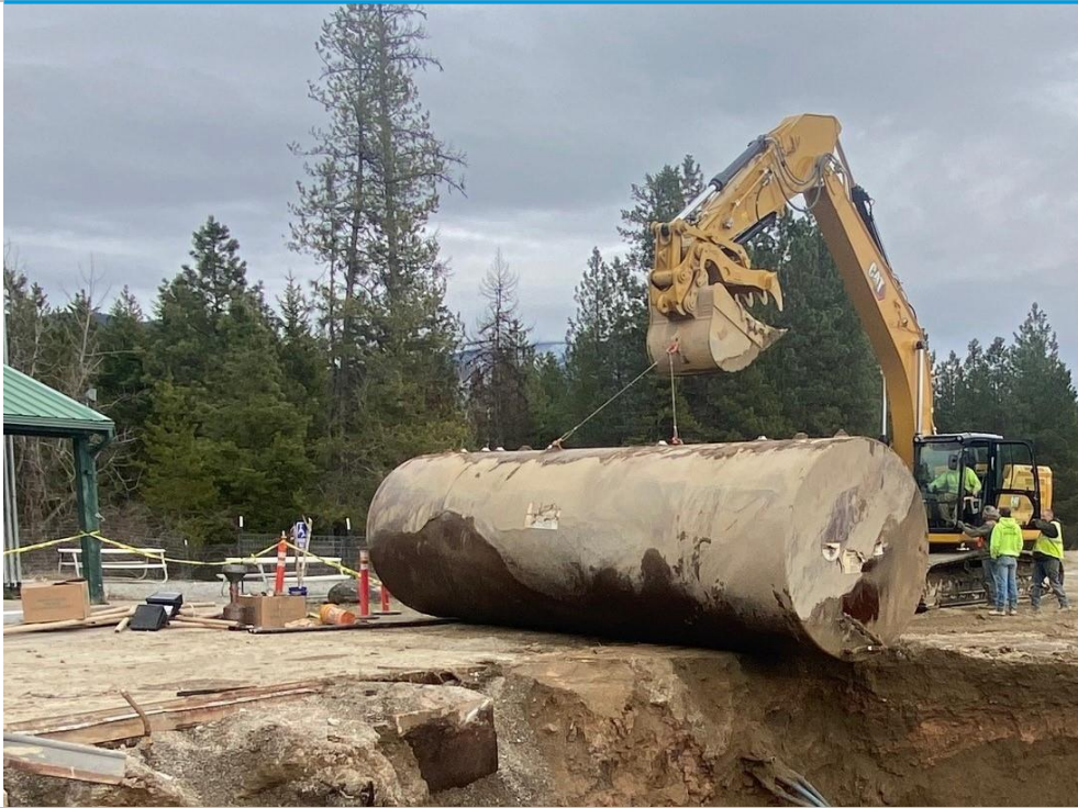
Removal of underground storage tank at Henry's Hideaway
