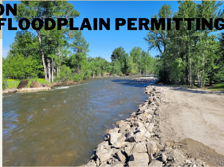
Riprap placed along the East Rosebud River bank after flooding and bridge repairs on Hwy 419 near Absarokee to restore access to Fishtail and Nye likely triggered emergency permitting. Photo by: S. Wingard (June 2022)
