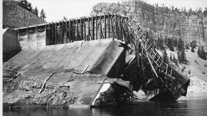
Above: The first Hauser Dam was one of only three steel dams in the world in 1908. As a result of the dam's failure, engineers saw the use of steel as a cautionary tale and no steel dam has been built since, even though the steel was not at fault.
