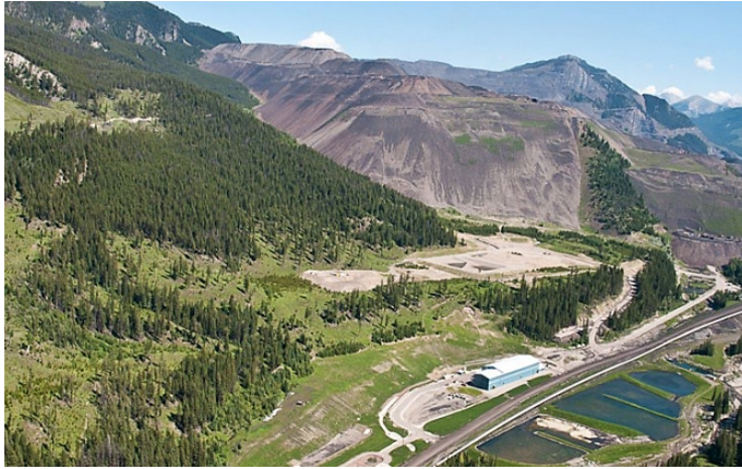
TECK RESOURCES WATER TREATMENT PLANT IN ELK VALLEY, B.C. (TECK RESOURCES)
