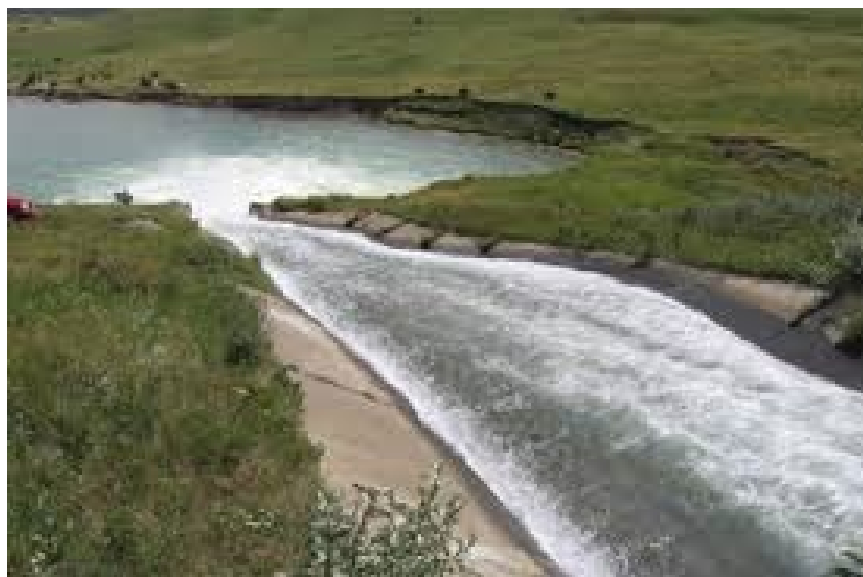
Figure 2 - St. Mary Diversion Pipeline and Drop Structure that provides water to the Milk River. The Milk River provides drinking water, irrigation water and recreation to hundreds of thousands of Montanans living along Montana's Hi-Line.
