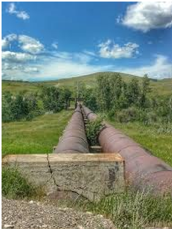
Figure 2 - St. Mary Diversion Pipeline and Drop Structure that provides water to the Milk River. The Milk River provides drinking water, irrigation water and recreation to hundreds of thousands of Montanans living along Montana's Hi-Line.
