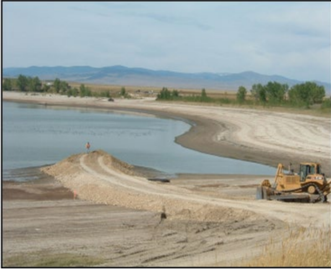
Figure 3 Ackley Lake Reservoir Cofferdam
