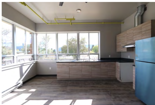
Figure 11 Interior renovation of hospital space to residential space at the Livingston Memorial Hospital. Photo credit: Homeword.
