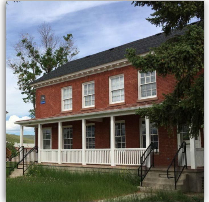
Fort Harrison Officer's Quarters, Helena | After Rehabilitation
