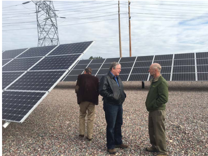
ETIC Chairman Keith Regier, right, visits with a representative of the Montana Electric Cooperatives' Association at the Flathead Electric Solar Utility Network community solar project near Kalispell.
