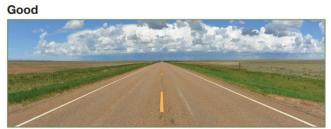
Visible traffic wear with low severity cracking and minimal rutting
