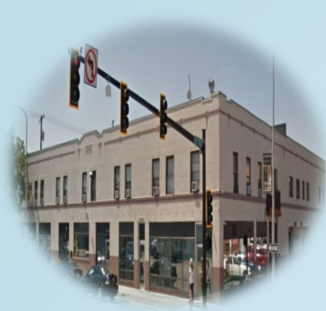
Alpha House Pre-Release Center
