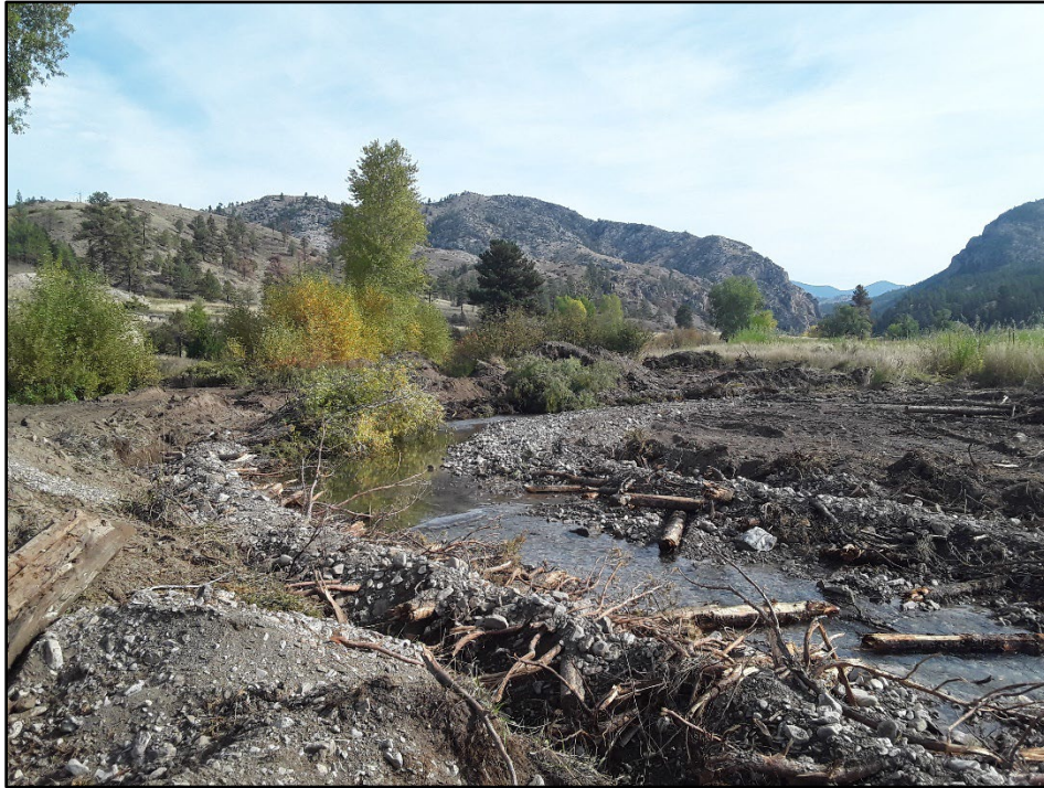
Figure 4. Top of the project area, station 47+00, open streambanks before willow placement.
