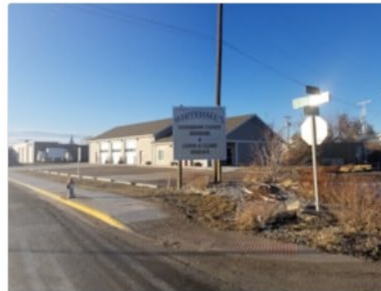
Whitehall Distribution System Improvements
