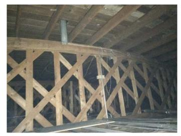
The Metals Technology Building was constructed in 1944 and is approximately 11,211 square feet. Lack of adequate attic insulation results in poor energy efficiency and increased utility costs. Roof truss support structures are showing signs of lateral stress. The roof membrane has blistering, wrinkles, and differential shrinkage which is causing leaking around the roof drains and flashing.
