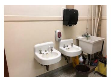
The restrooms are small, outdated and not ADA accessible. Many have not had significant improvements since the buildings were constructed. A complete renovation will remove everything down to the structure. Where possible, restrooms will be expanded and made accessible. New plumbing, fixtures, flooring, partitions, and lighting will be installed.
