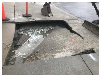
The current water main loop system connects all main campus buildings and when a break occurs, the city main must be shut off resulting in loss of water at every building. The water pipes are beginning to fail causing damage to buildings and infrastructure. In 2020, a pinhole sized pipe failure outside McMullen Hall caused \$35,000 of damage. A pipe failure in September 2021
