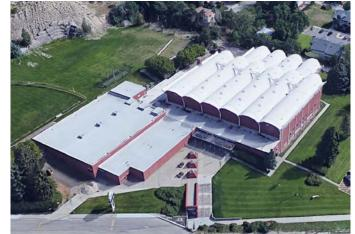
The roof was last replaced in 1992 and is well past its expected useful life. Repairs of approximately \$50,000 and annual maintenance of \$15,000 will extend the life of the roof until 2023. The roof is leaking, causing internal damage to the P.E. Building. RMTD will no longer cover internal damage as it is caused from deterioration and not a destructive event. All sections of the curve and flat roof are due for replacement.
