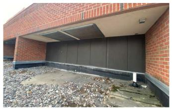
Tietz Hall has a single ply, ballasted roof that is original to the facility and well beyond its expected useful life. The roof protects expensive mechanical equipment that researchers rely on for the continuity of their work. Failure of the roof system causing damage to the mechanical equipment and disruption of controlled environments has the potential to cause significant damage to Animal Resource Center research operations.
