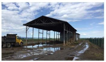
The BART Farm Hay Shed Building #455 is also no longer in use due to its physical condition and will be demolished. In addition, structural deficiencies in Hay Shed Building #456 will be addressed to remedy immediate life-safety concerns. If not addressed, common conditions like high winds or snow loads could cause the buildings to collapse.
