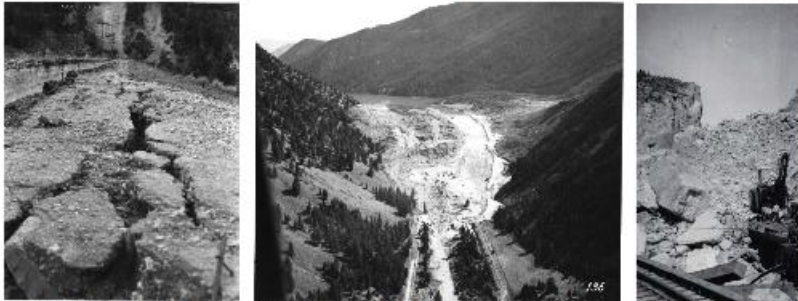
The historic magnitude 7.3 earthquake at Hebgen Lake on August 17, 1959 caused cracking and slumping at the crest of Hebgen Dam (left). The Madison Slide (center) killed 25 people where it dammed the Madison River to form Earthquake Lake. The 1925 Clarkston Valley earthquake triggered the Deer Park slide (right) and extensively damaged schools, churches, and railroads in Three Forks and Manhattan.
