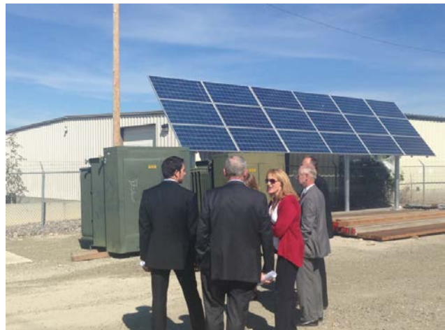
Members of the ETIC visit NorthWestern Energy's Battery Storage Project in Helena during a Sept. 2015 meeting.
