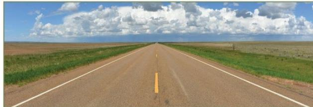
Visible traffic wear with low severity cracking and minimal rutting
