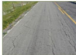
Prevalent cracking in extent and severity, heavy rutting, patching
