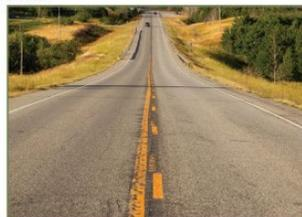
Moderate cracking in extent and severity, slight rutting and aggregate loss
